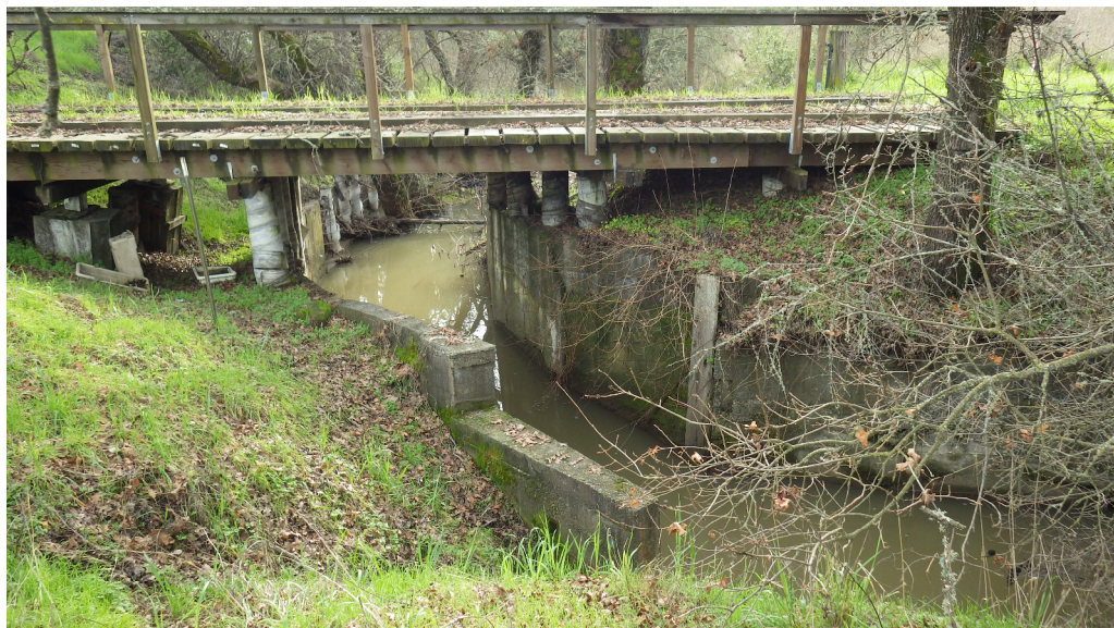
Image 3. Existing View of Bridge
