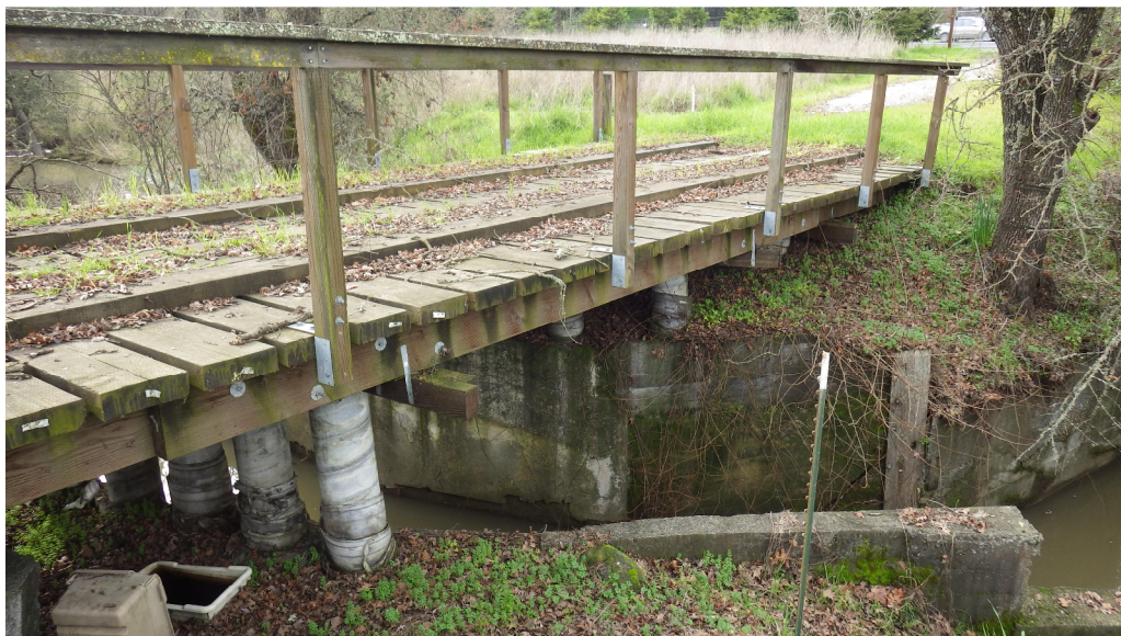
Image 2. Existing View of Bridge
