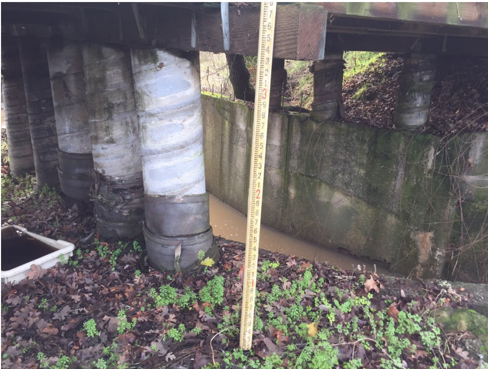
Concrete support posts and most concrete revetment walls will be lifted and removed from the bed and banks taking care not to allow rubble or detritus from entering the channel cross section as fill.
