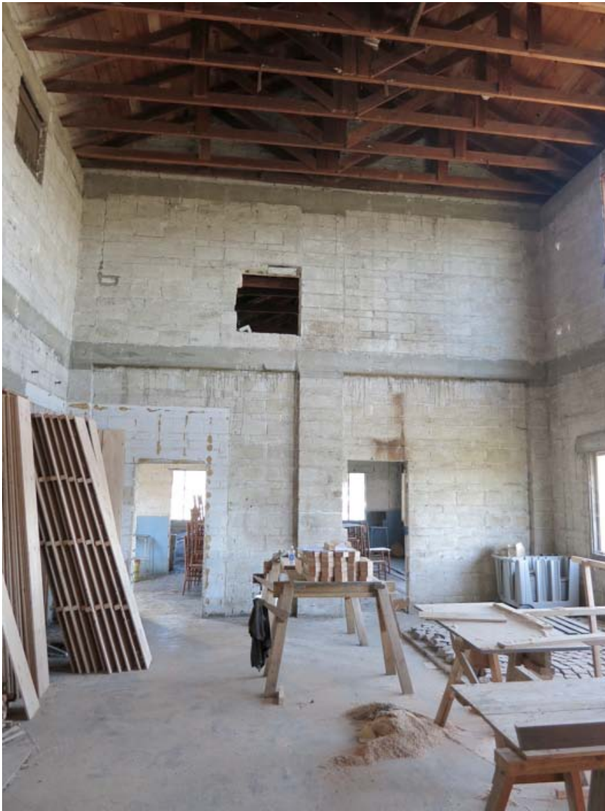
Interior of central two-story section. Note that only the structural blocks rafters and roof remain. All of the finishes are missing including the balcony, stairs and ceiling as well as mechanical and electrical systems.
