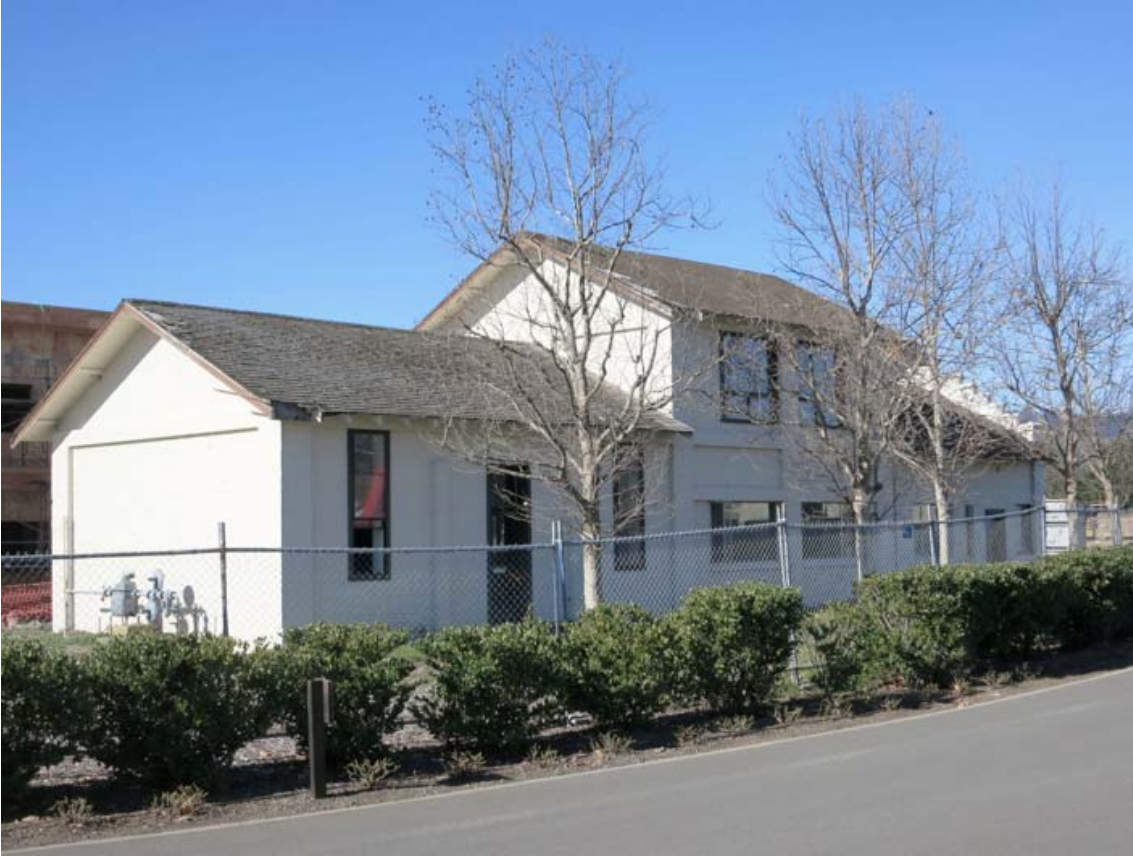
Exterior View looking northwest. Note that all historic windows and doors are missing as well as stucco finishes and the roofing is in very poor condition.
