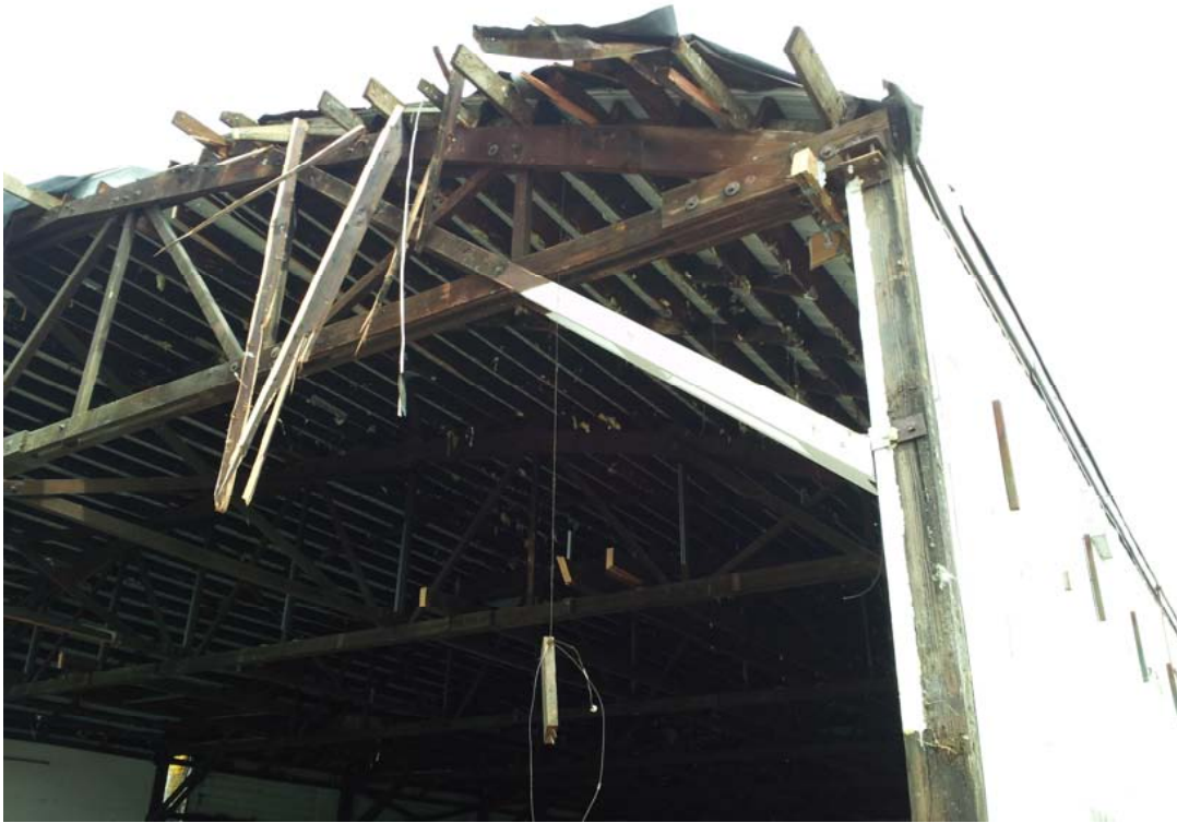
Detail of Forni-Williamson trusses.
