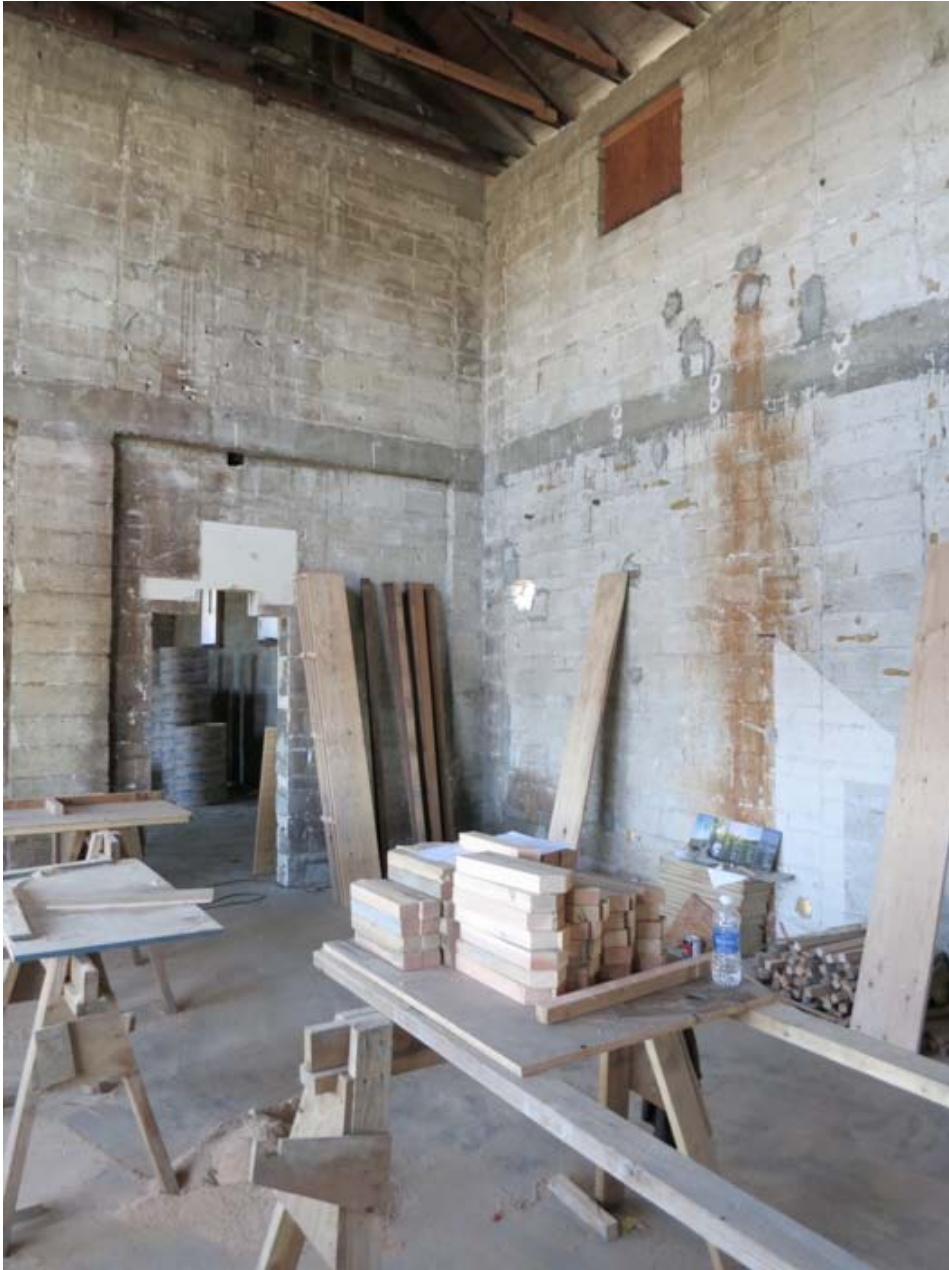
Interior view of central two-story section. Note all finishes are missing. Scar trace of stairs to the second floor are visible on the right wall.
