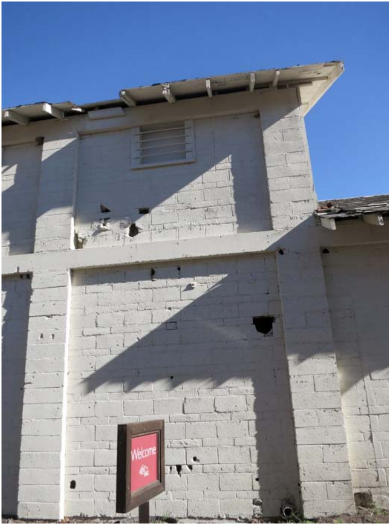
Exterior Detail of west two-story section. Note damaged block wall and missing exterior stucco finishes.
