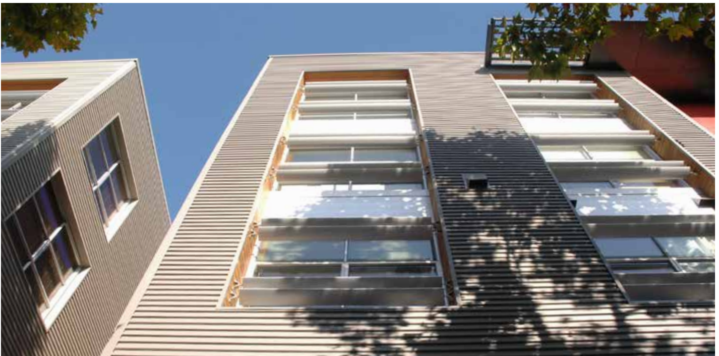
Figure 5.15 Deep awning, recessed windows, deep window louvers, and overall material texture all contribute to create depth and shadow that modulate the façade.
