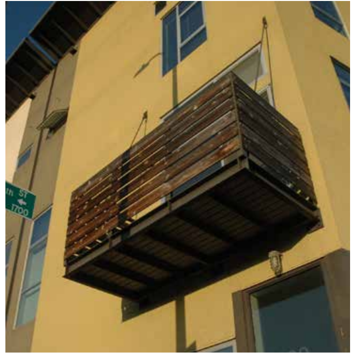
Figure 5.13 Well-detailed steel and wood hanging balconies with attention to the method of joinery.
