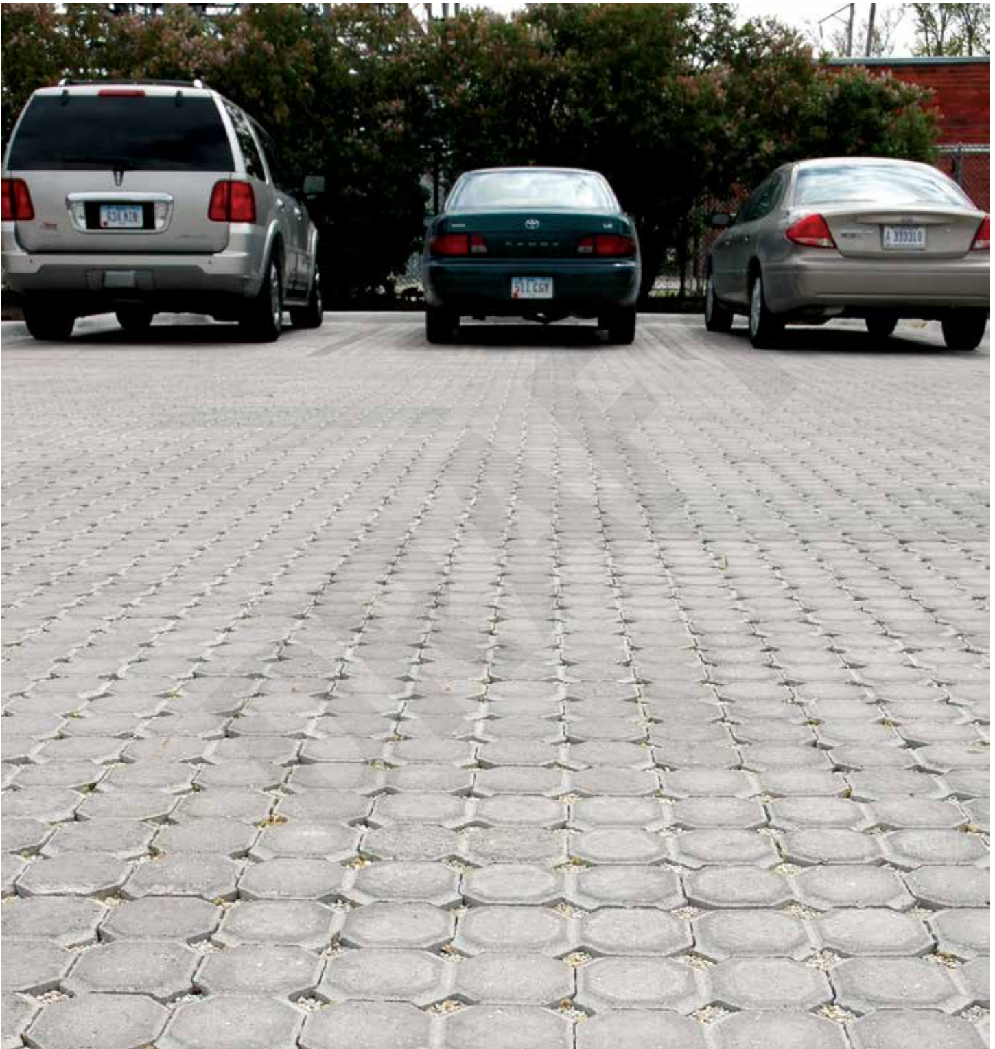
Figure 6.8 Permeable paving for parking areas reduces stormwater, increases groundwater recharge, and has attractive texture.
