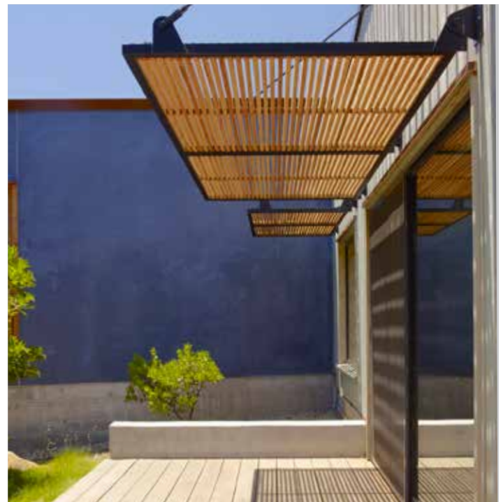
Figure 5.13 Well-detailed open deck with slatted wood shading system and attention to the method of joinery.
