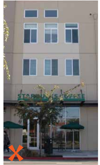
Figure 5.15 Bad: Building walls are too planar and have poor thickness and visual character due to insufficient window reveal and insufficient depth of articulation.
