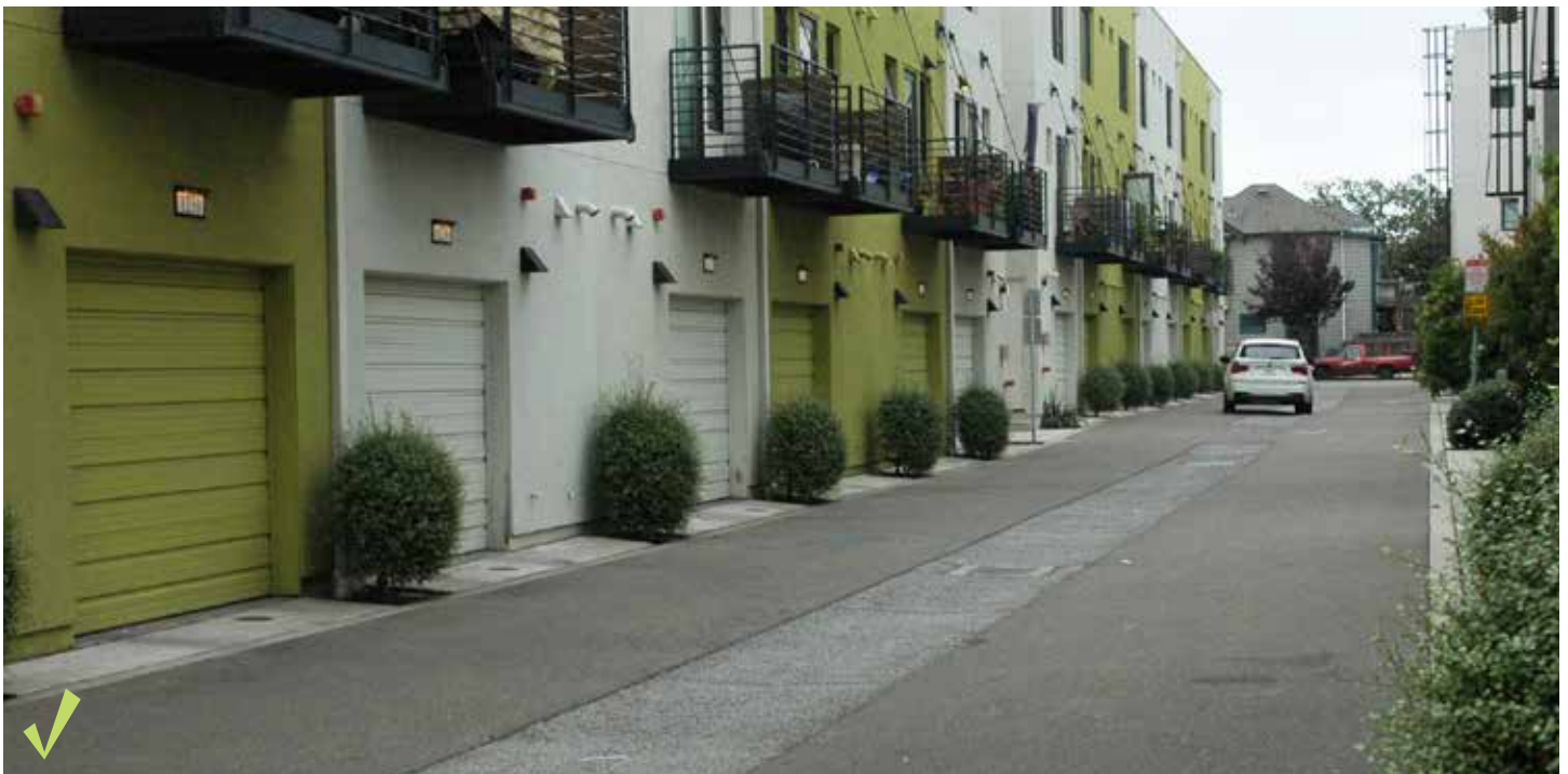
Figure 5.15 Good: Garage door openings are recessed at least 1' from the facade plane, a maximum of 9' high.
