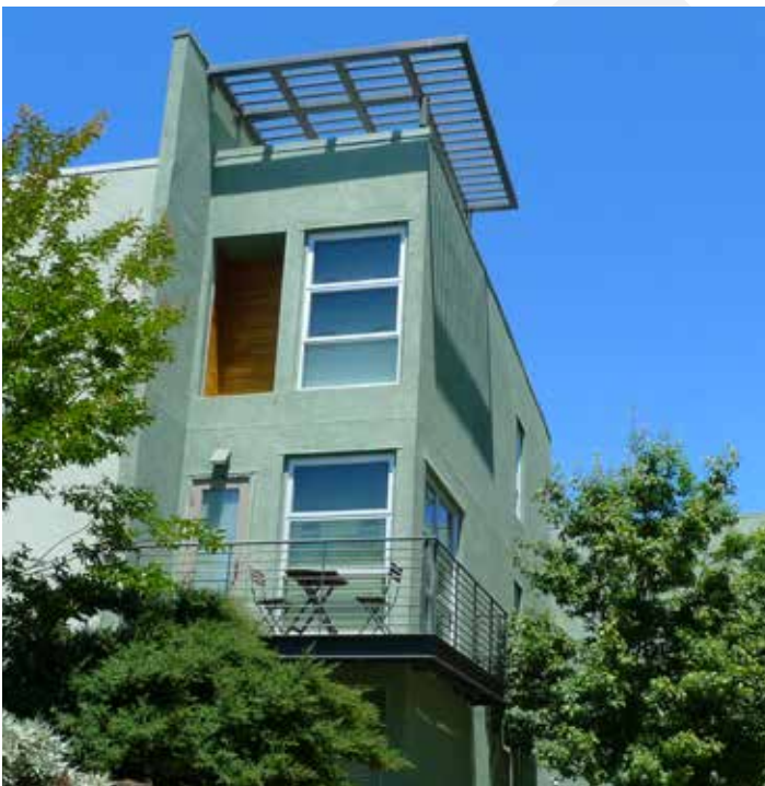
Figure 4.35 Simple, metal frame windows recessed from the facade plane
