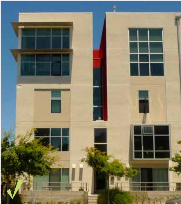
Figure 5.15 Good: Building wall has perceivable thickness with window reveals, projections, deep recesses, and overhangs.
