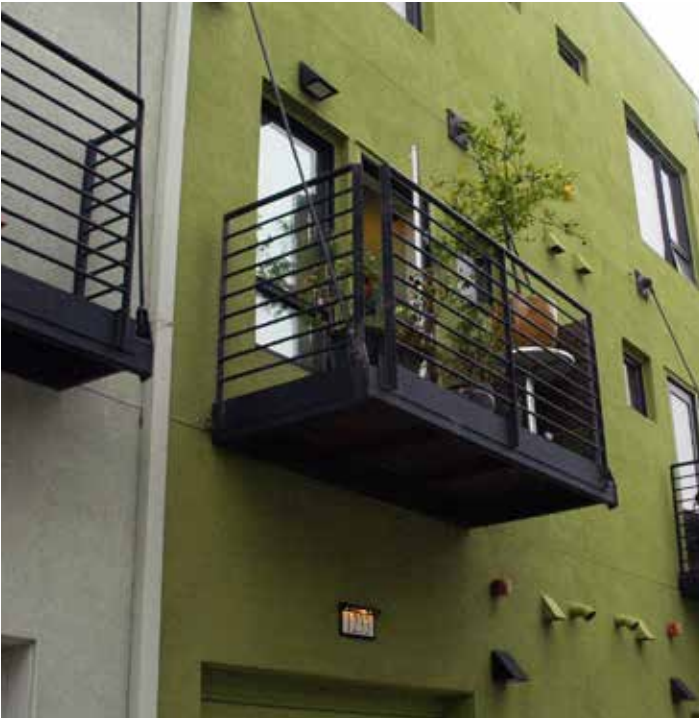
Figure 5.13 Well-detailed steel and wood hanging balconies with attention to the method of joinery.
