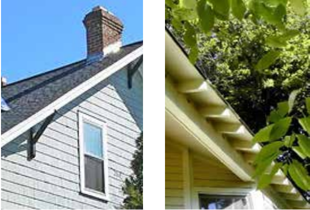
Figure 4.23 Eave with knee bracket (left) and rafter tail (right)
