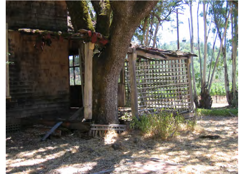
Porch collapsing around existing tree
