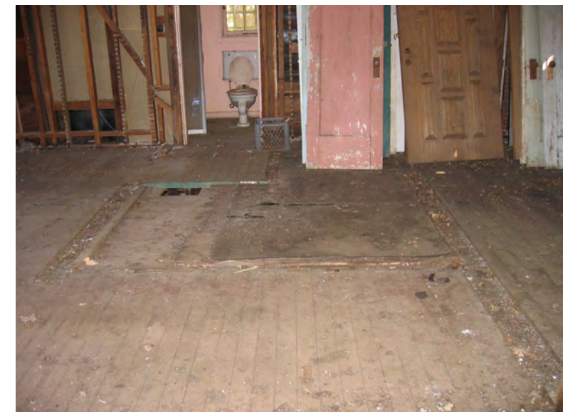
Interior wall layout evident in finish floor
