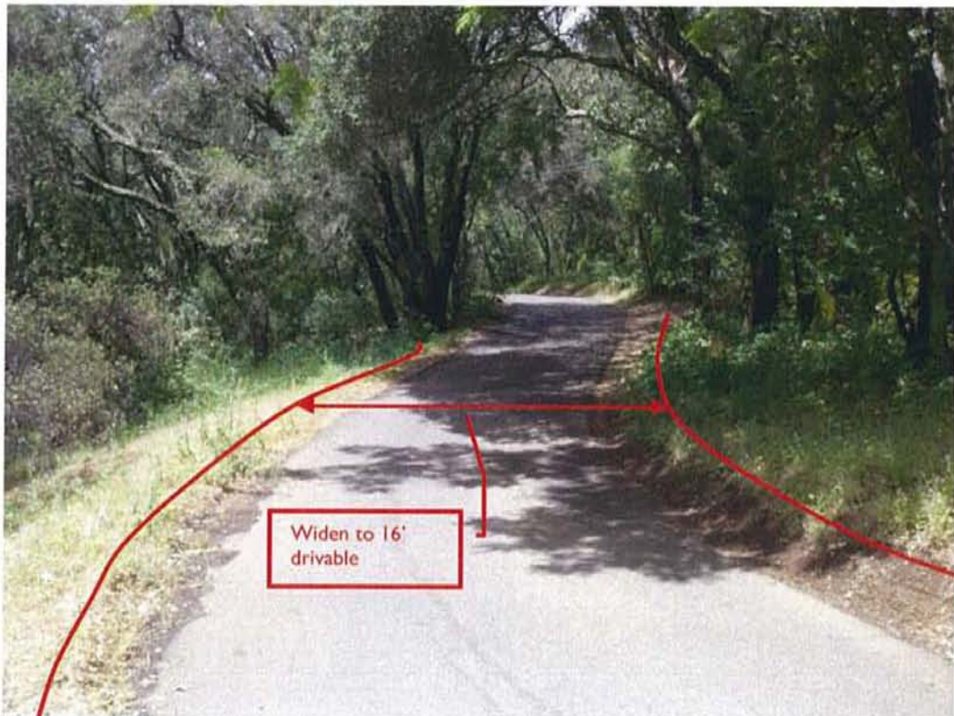
Photograph looking north along existing driveway alignment at STA 501+10 Reduced width to allow preservation of steep slopes (left) and native trees
