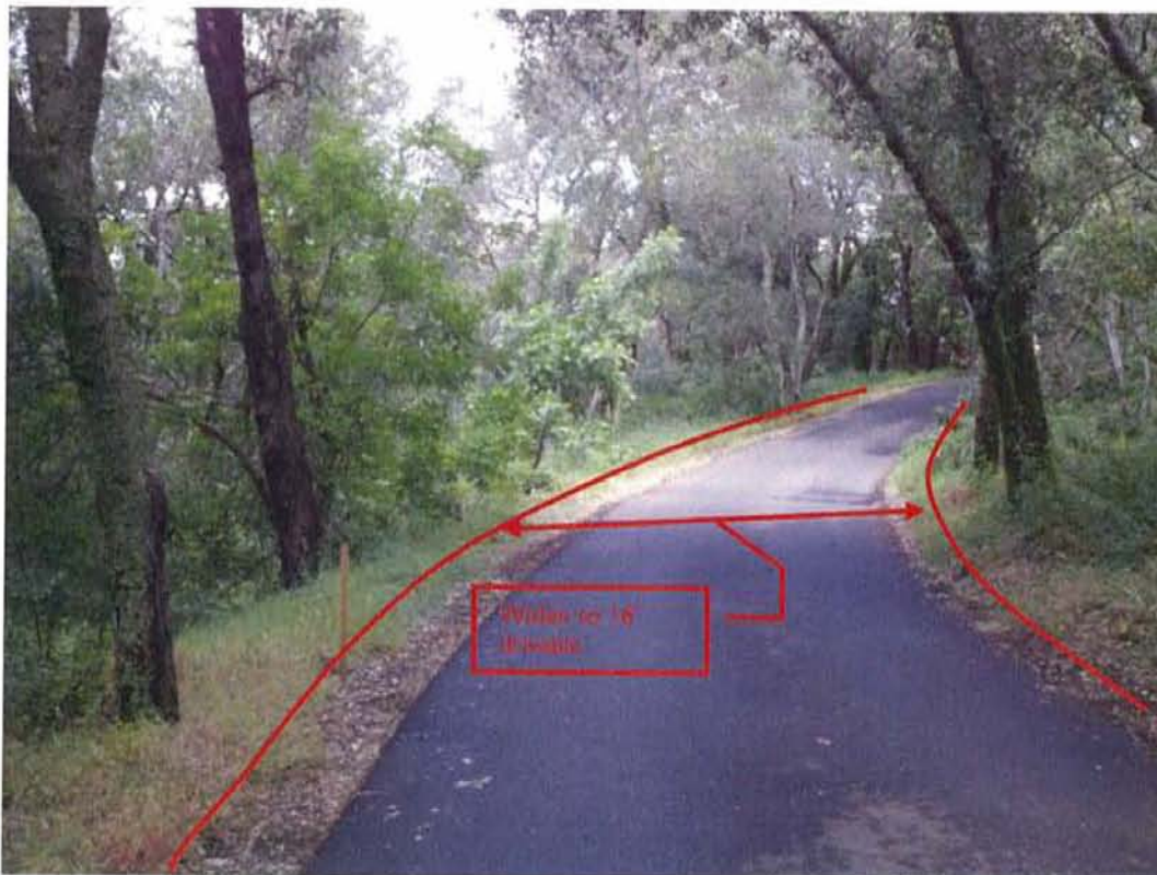
Photograph looking northeast from STA 507+50 Reduced width will allow preservation of slopes (left) and native trees
