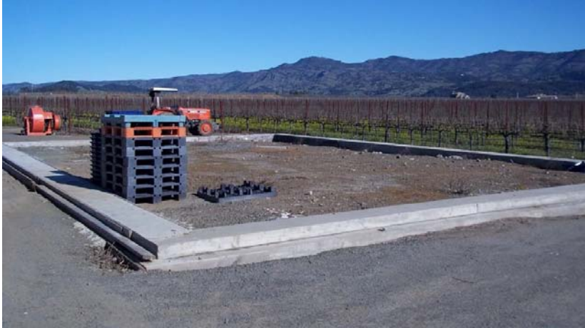
Existing barrel building foundation
