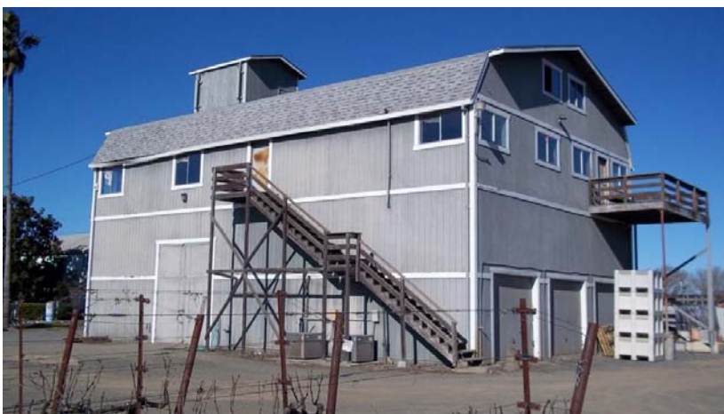
Existing winery barn
