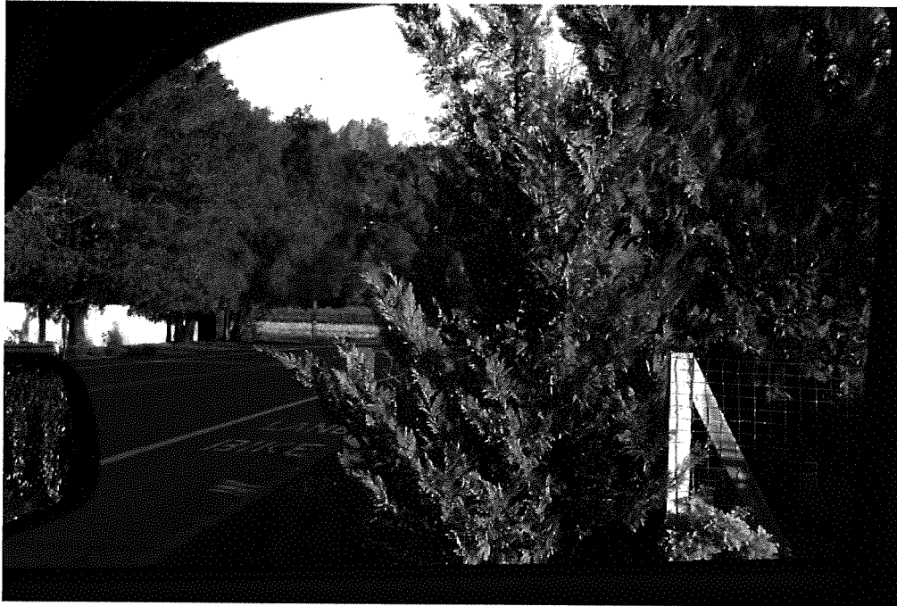
Photograph 1: View to south from existing driveway at Silverado Trail illustrating reduced sight distance due to vegetation (December 16, 2008)
