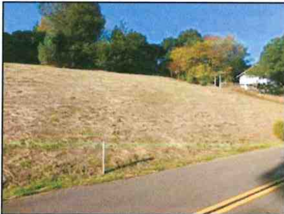
Empty lot across from 318 Circle Oaks Drive. The house formerly on this lot had to be demolished after heavy rains caused foundation shifts. The land was then extensively re-graded and drains installed.
