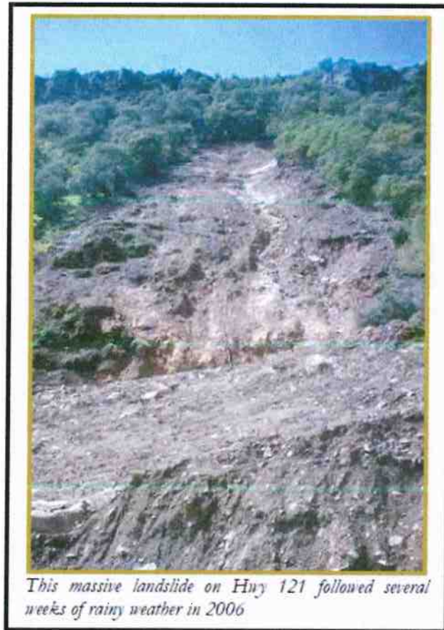
Above: January 2006 landslide on Highway 121 , photo from the General Plan, p. SAF-2
