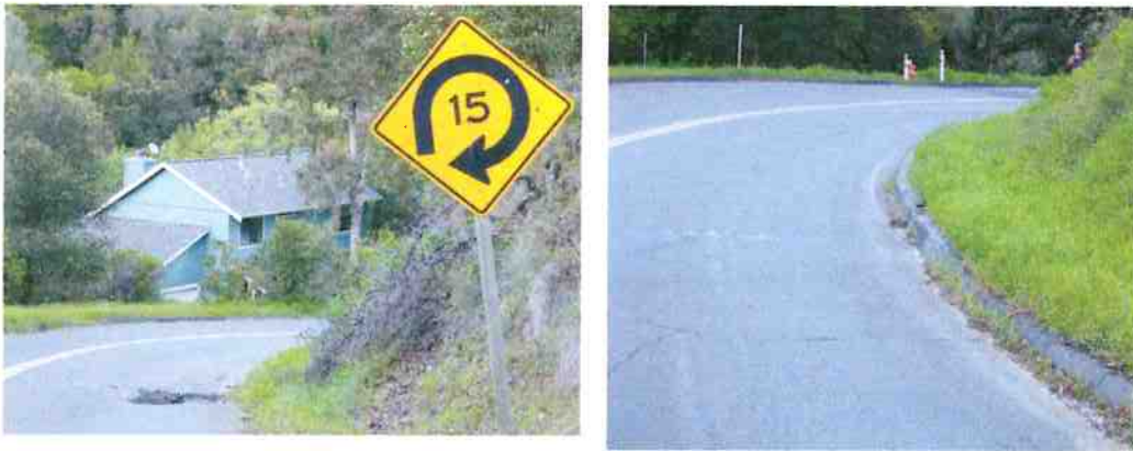
Pictures illustrating blind curves, short lines of sight on steep grade of Circle Oaks Drive. The house visible on the left is at 218 Circle Oaks Drive.
