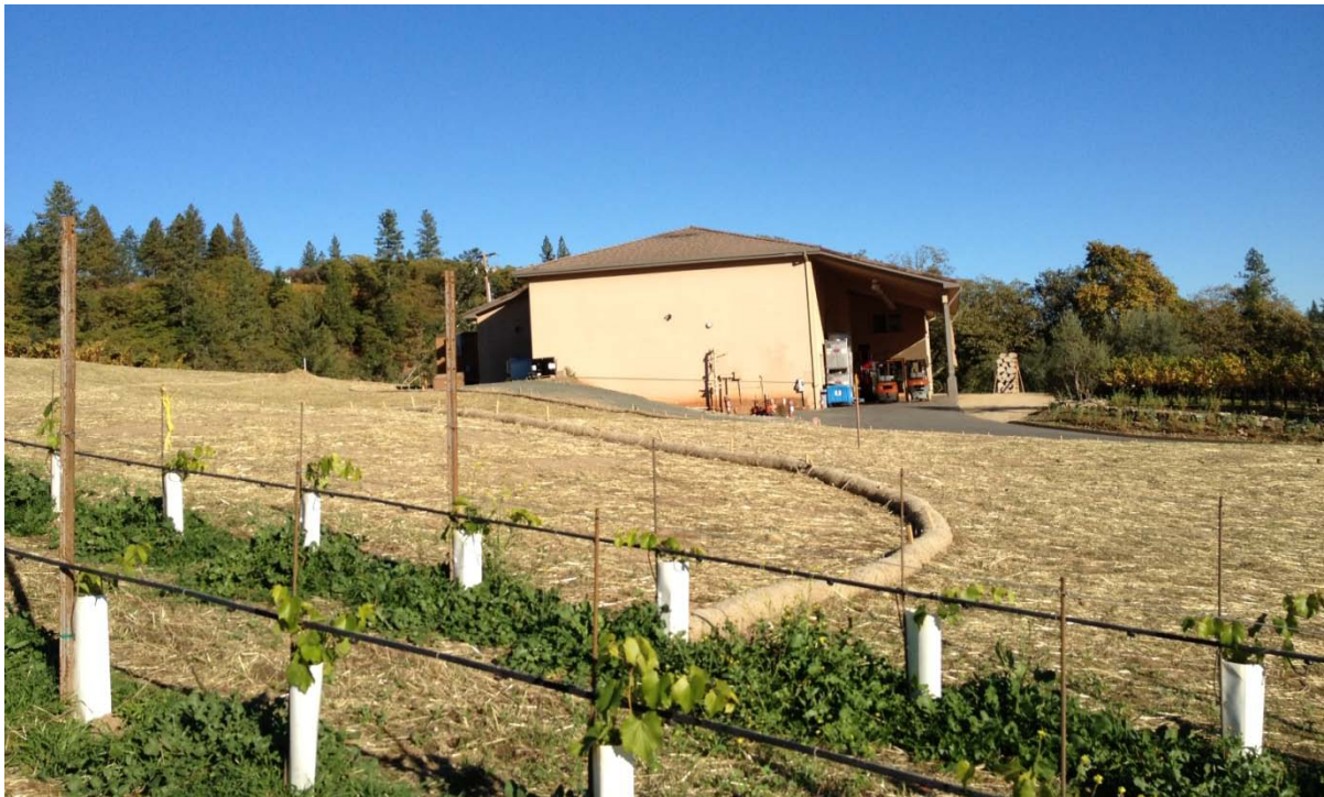
Existing Winery Building
